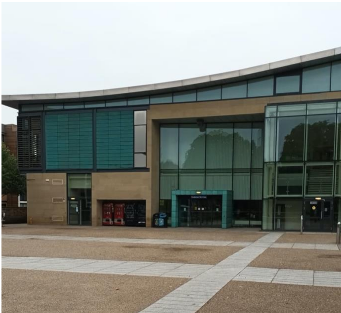
Entrance to the Edge from the car park end for Customer Services Desk (Endcliffe Student Room check in/out)
